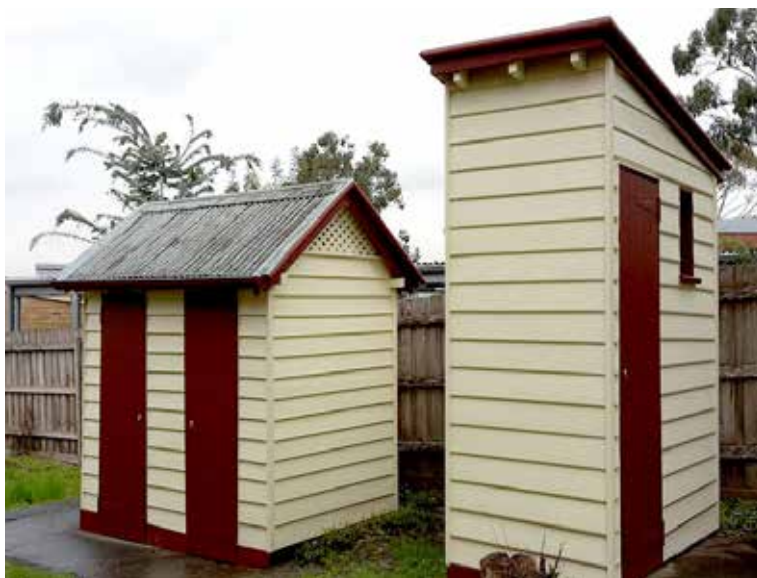
Yarra Ranges Council contractors have repaired and painted the former toilets behind the court house. They will now last for a long time more.
